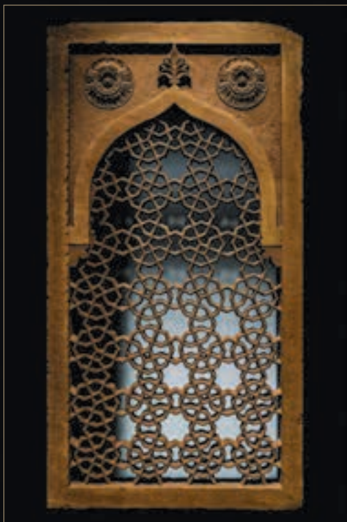
An example of a jali in Indian architecture. Photo © Sylvain Collet/Bridgeman Images
