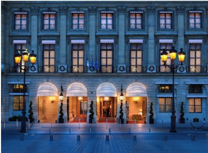
Facade of the Ritz Paris, prior to the renovations
