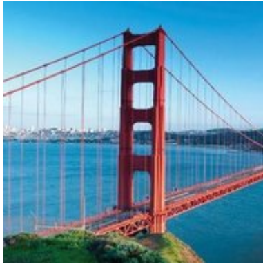
Golden Gate Bridge
