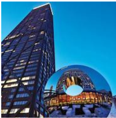
Exterior image of The Ritz-Carlton, Chicago
