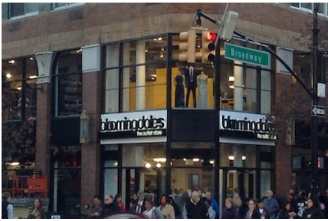
Exterior of Bloomingdale's Upper West Side Outlet
