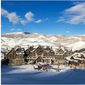
Exterior of The Ritz-Carlton, Bachelor Gulch
