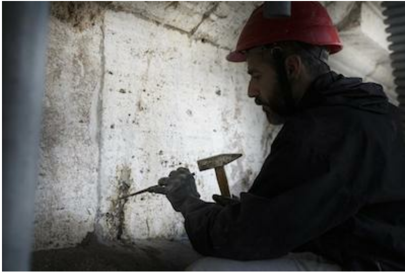
Worker on-site at the Colosseum
