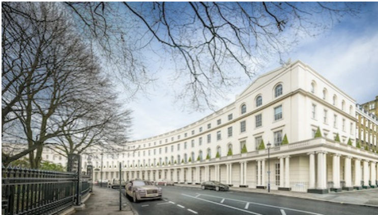
Park Crescent overlooking Regent's Park, London
