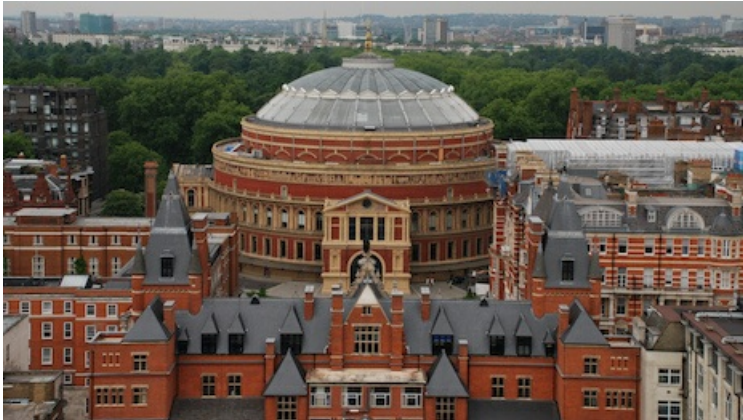
London's Royal Albert Hall, photo courtesy of Harrods Estates
