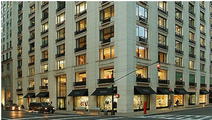
Exterior of Barneys New York flagship. Image credit: Barneys
