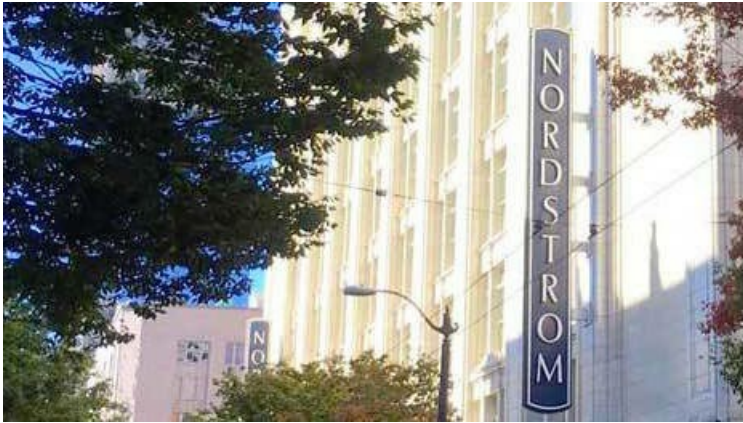
Exterior of Nordstrom's Seattle flagship store. Image credit: Nordstrom
