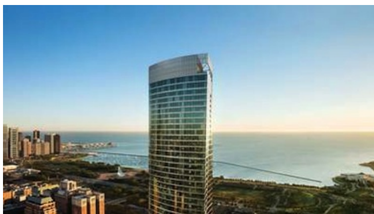
Chicago's 1000M is located on one of the city's most iconic streets
