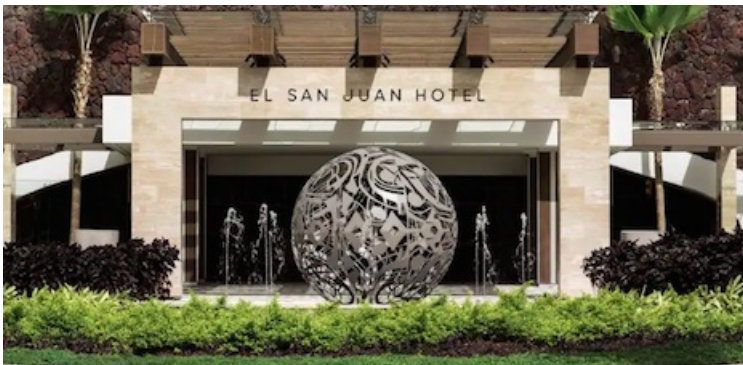
El San Juan Hotel in Puerto Rico. Image credit: Hilton Hotels
