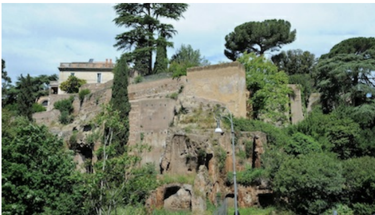
Gucci is working to restore the Rupe Tappea in Rome. Image courtesy of Gucci
