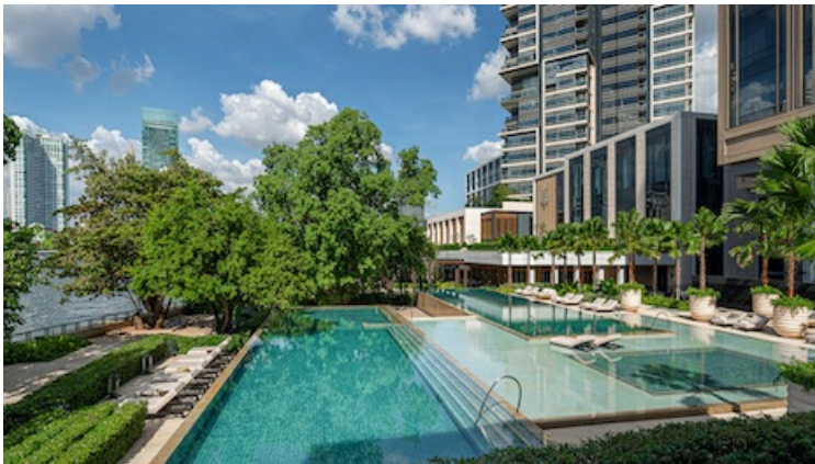
The riverside infinity pool at Four Seasons Hotel Bangkok at Chao Phraya River. Image credit: Four Seasons
