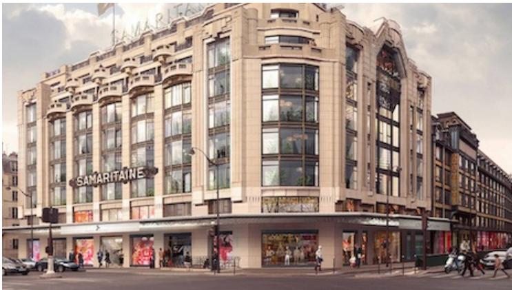
From quai du Louvre, rendered view of the Cheval Blanc hotel. Image credit: LVMH
