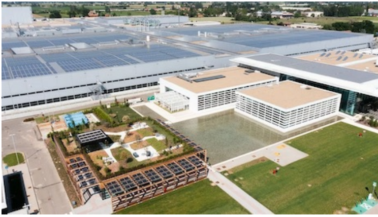
The Philip Morris International production facility will get one step closer to decarbonization thanks to the venture. Image credit: Ferrari
