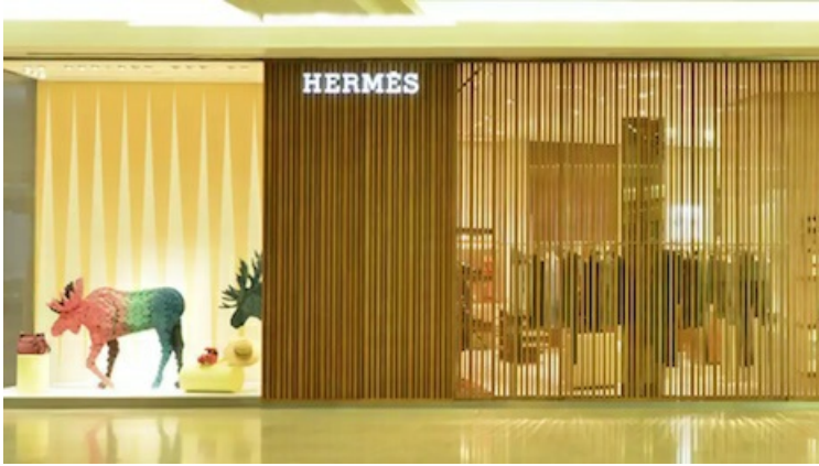
The Malaysian store's facade is made of woven bamboo and cane. Image credit: Herms
