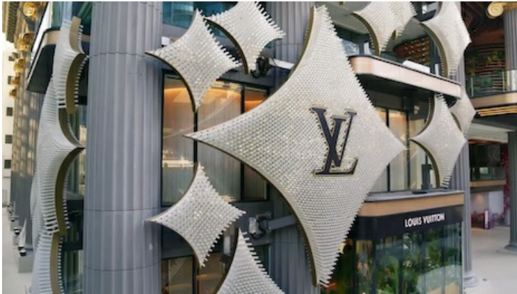
The opening is referred to as LV The Place Bangkok. Image credit: Louis Vuitton
