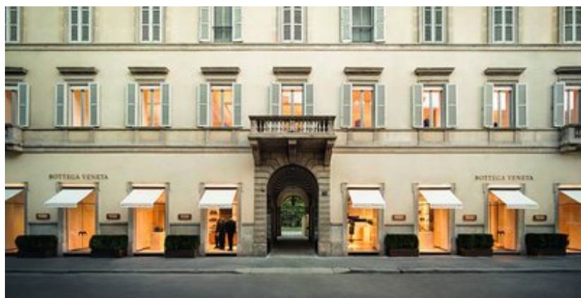
Exterior of Bottega Veneta's first maison
